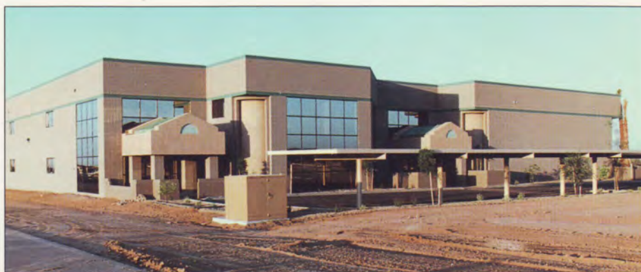
Above: The headquarters of Data Sales Co., located in Burnsville, Minnesota Below: Scottsdale, Arizona location
